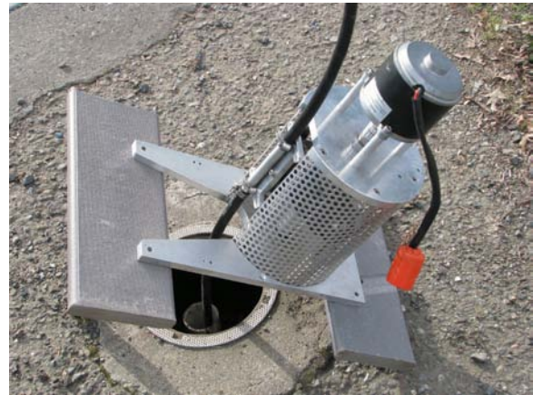
Pump rotated down onto well for pumping.
